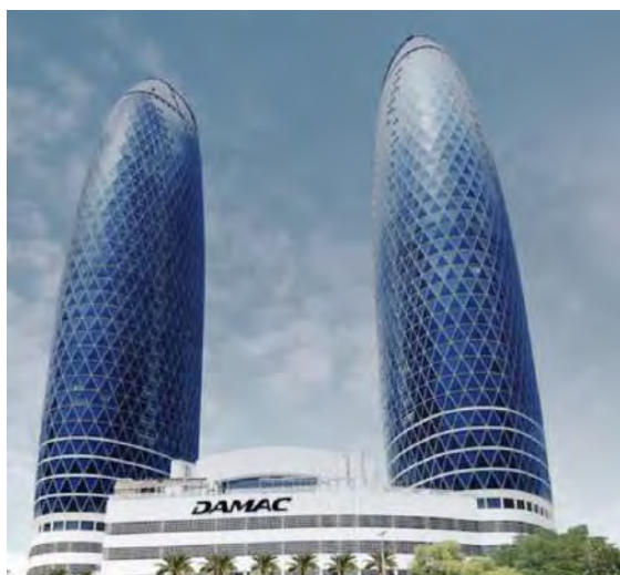
Park Towers at DIFC 1 Dubai, UAE
