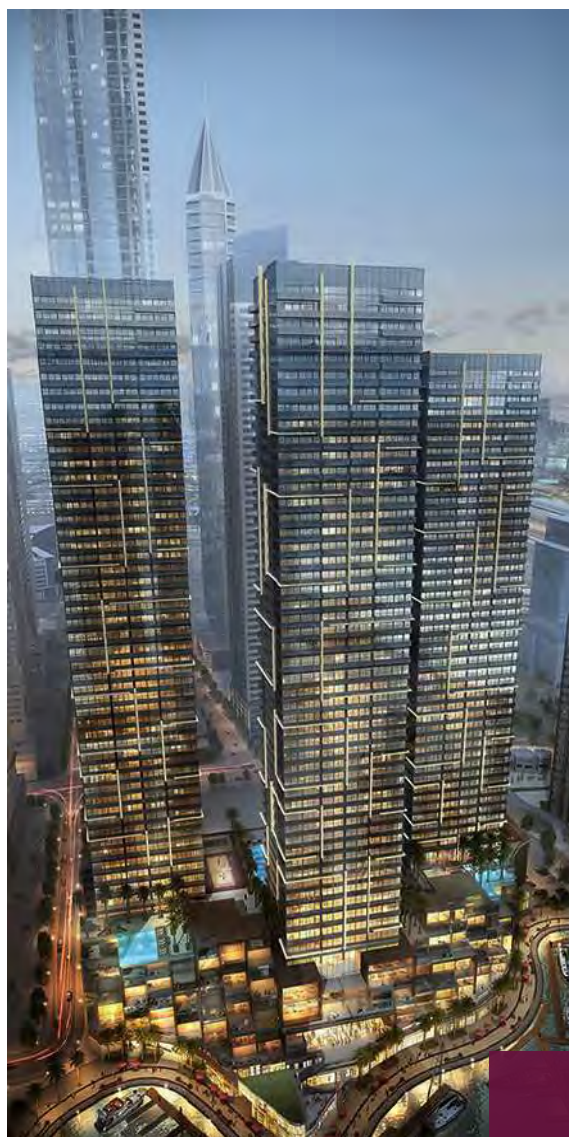
Marina Gate 1 & 2 3 Dubai, UAE
